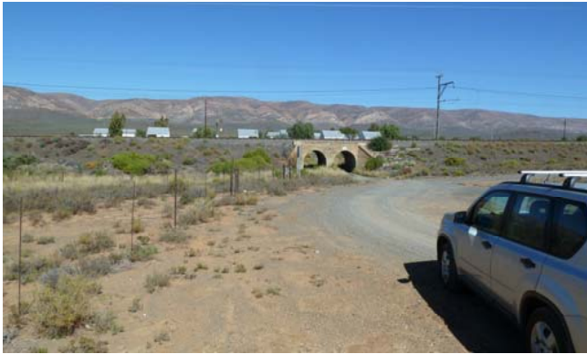
i. Vehicle underpass between north and south section of village
