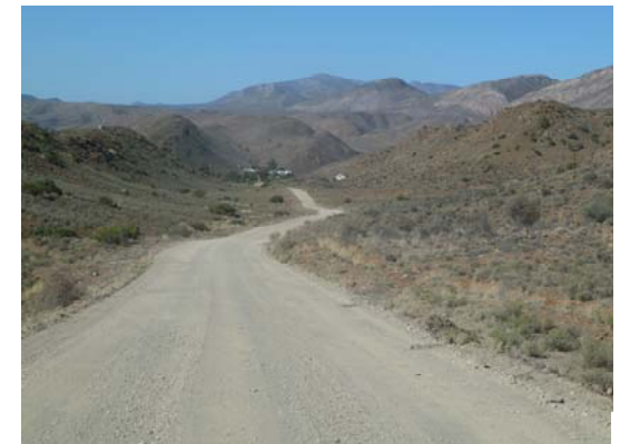
Photo 5.9 Roads requiring upgrading
