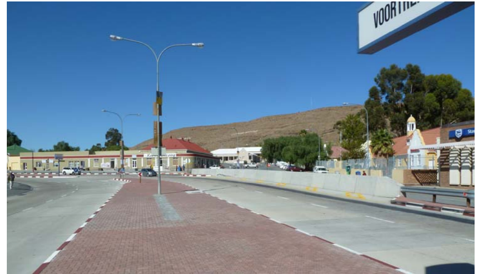
Photo 3.4.7.1 Barriers in the middle of town
