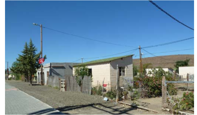
k. RDP houses in Bergsig West
