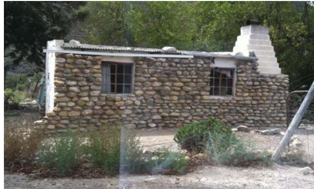
b. Historic stone-faced house in Vleiland
