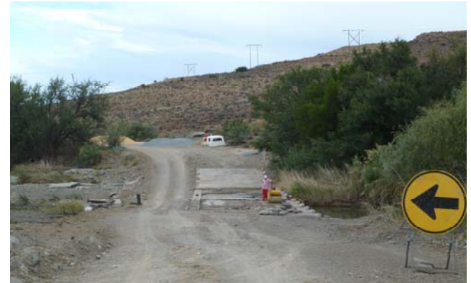
e. Bridge maintenance
