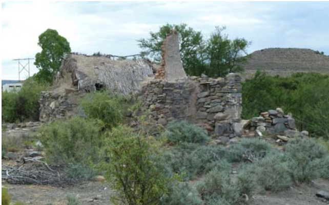
f. Ruined cottages at Koringplaas
