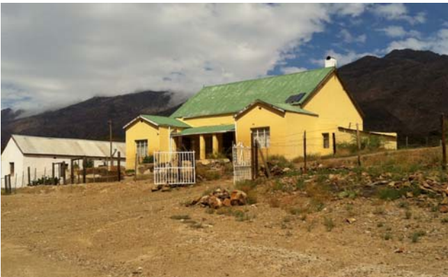
f. Houses in Vleiland
