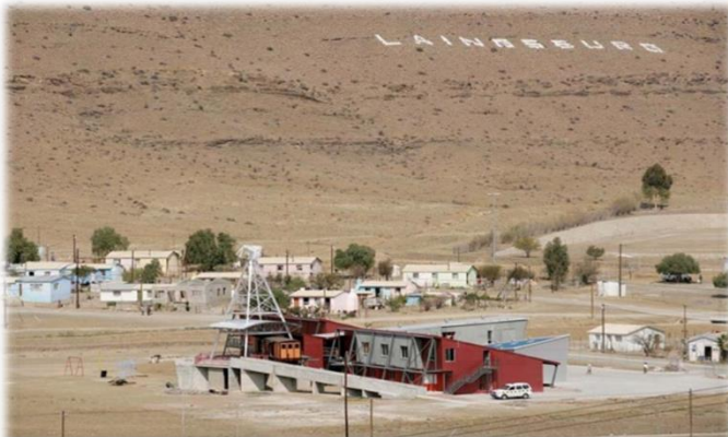
Laingsburg Multi-Purpose Centre, Laingsburg, Western Cape 2004. View from national road of building in it's context.
